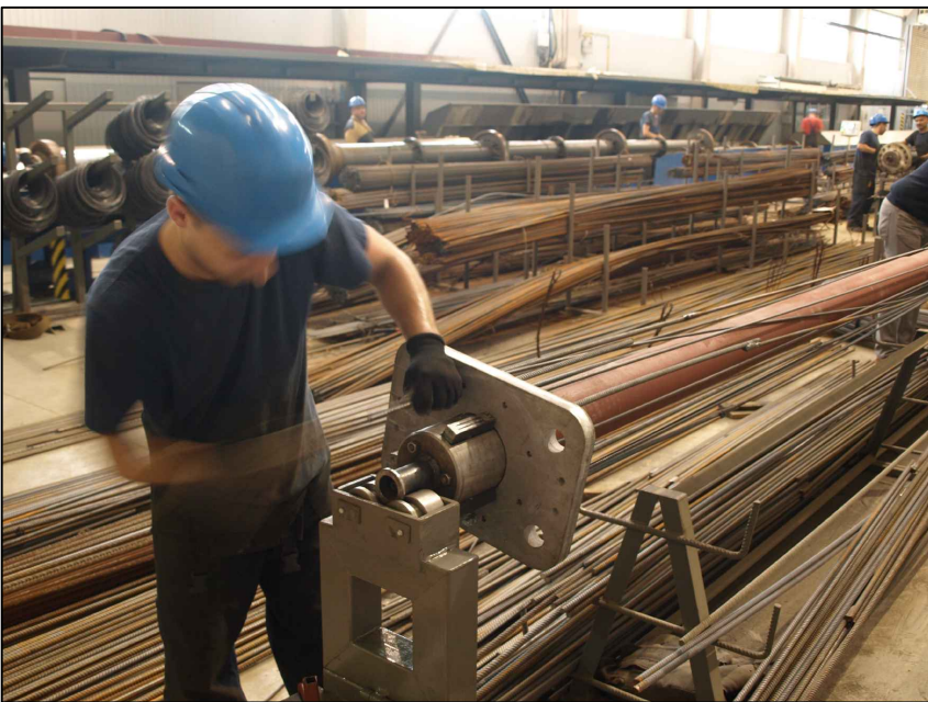
Fig.3. Construction of a reinforcement cage: phase 1 - moving the upset tendons through the head
