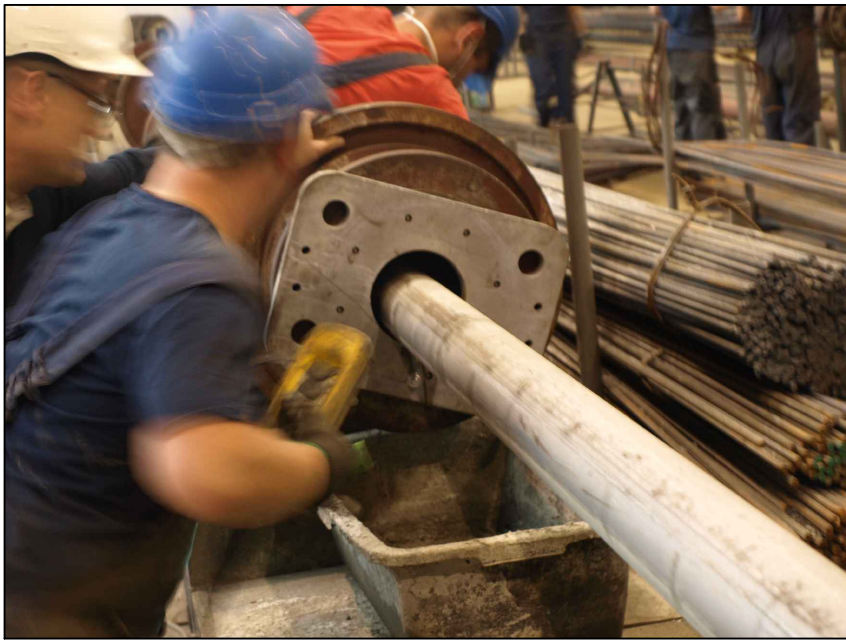
Fig.6. Introduction of the concrete mixture into the mold
